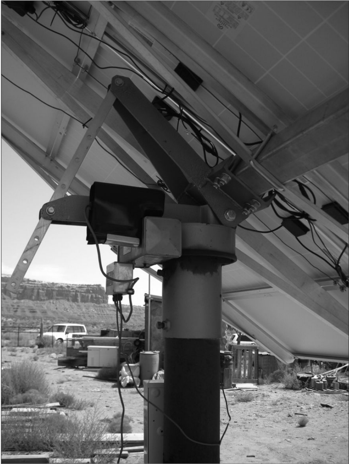
Adjustable head for pole-mounting of solar panel.
